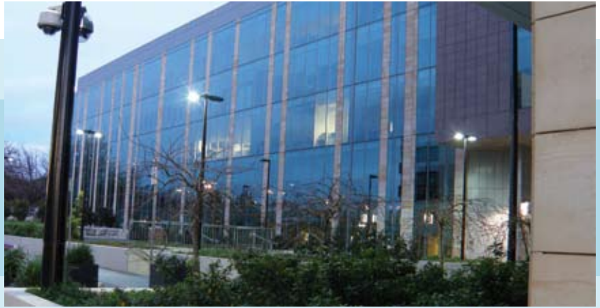
Figure 8.10: National Australian Built Environment Rating System (NABERS) for One National Circuit, Barton
